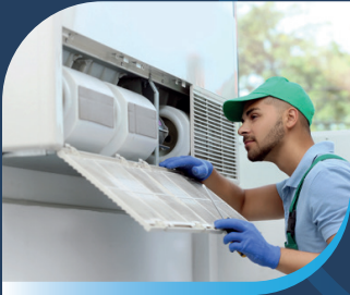
Air-Conditioning, Ventilations & Air Filtration Systems Installation & Maintenance
